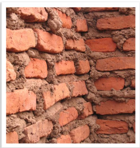
FIGURE 8: TRADITIONAL BRICKS IN MALAWI
