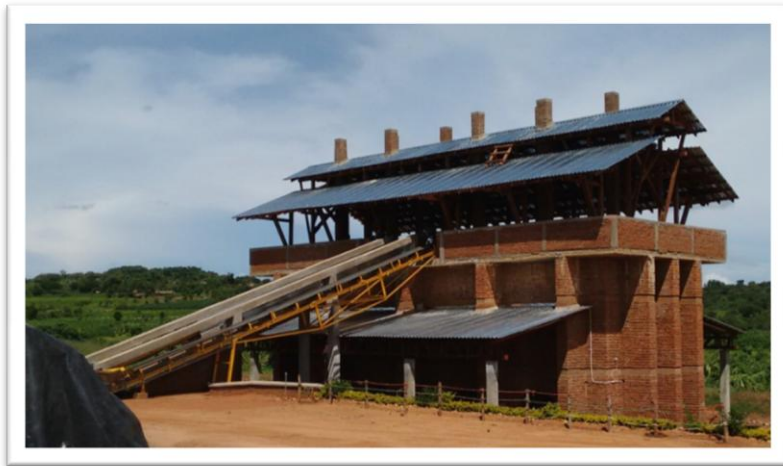
FIGURE 11: THE VERTICAL SHAFT BRICK KILN
