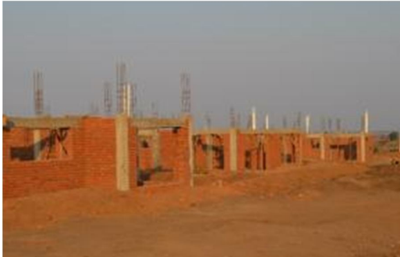
Figure 6: VSBK bricks being used in housing construction
