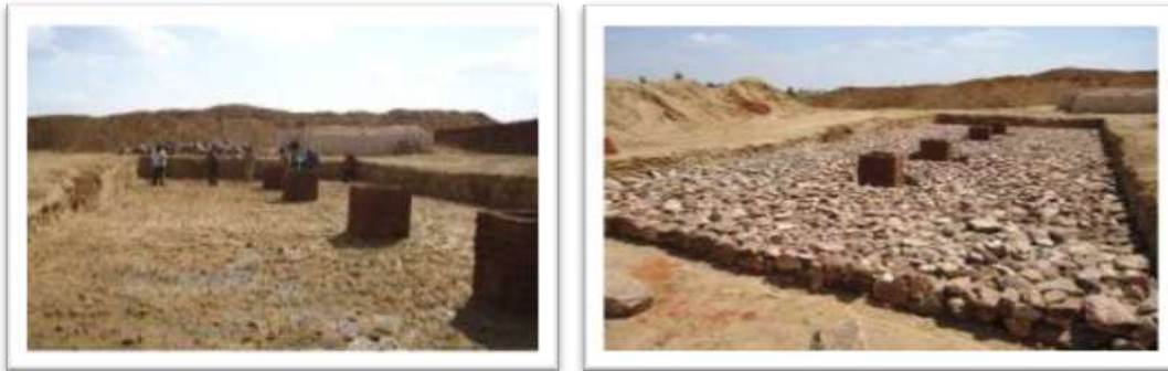
Figure 10 : Stone soiling
