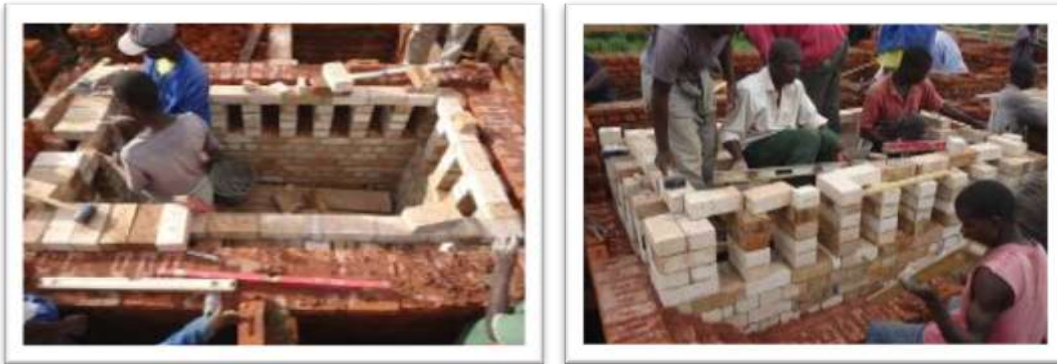
Figure 15 : Building the flue duct
