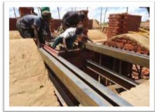
Figure 12: Setting C-channel
