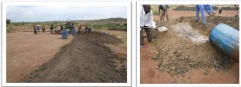
Figure 19: Dumped soil for ageing (left), Aging of soil (right)
