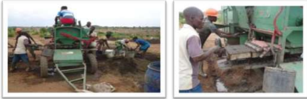
Figure 20: Mechanical Brick Moulding
