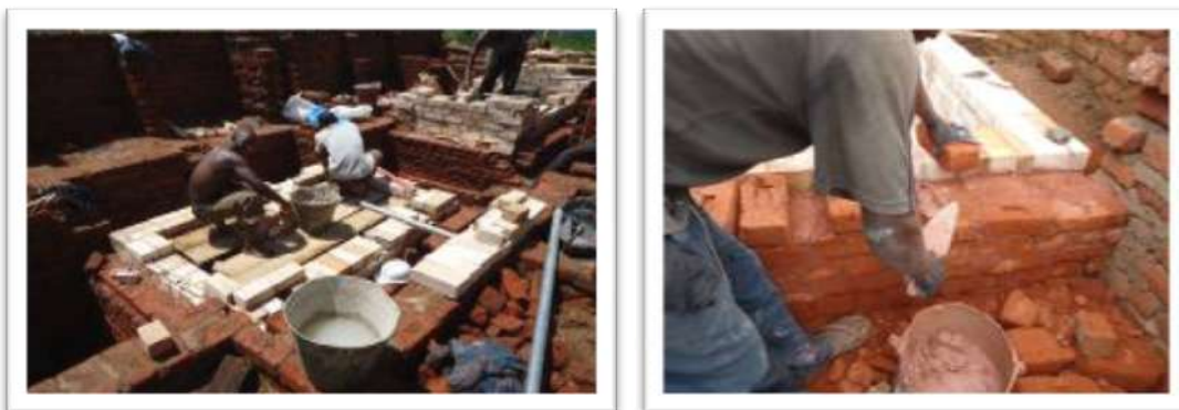
Figure 14: Dry refractory brick layers
