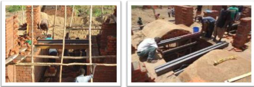
Figure 11: Setting I - Beam
