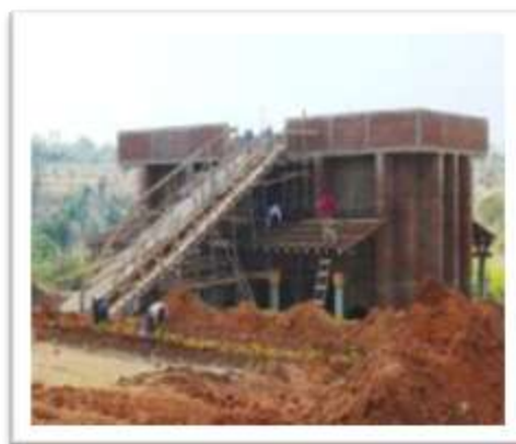
Figure 2: The VSBK under construction
