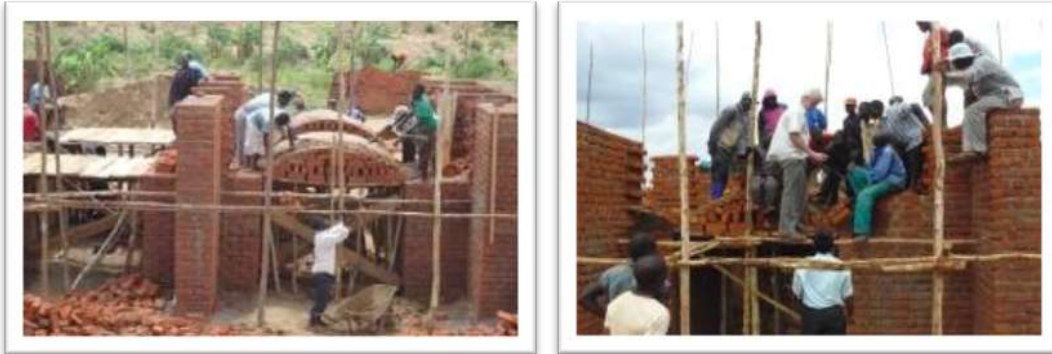
Figure 13 : Constructing brick arch
