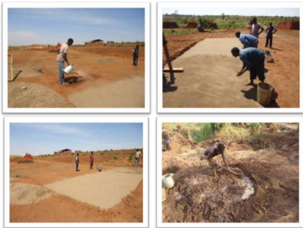
Figure 3: Watering leveled moulding yard (top left); Spraying sand over levelled and watered surface (top right); Proper moulding yard (bottom left); Aging of soil and manual mixing for appropriate soil mixture (bottom right)
